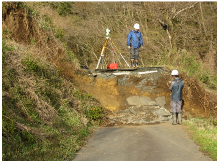
Photo 2: Fukushima-ken Hamadori earthquake (M 7.0) on 11 April 2011, accompanied by the significant surface faulting of normal fault-type.
